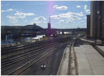
Railroad Infrastructure along the Mississippi River of St. Paul
